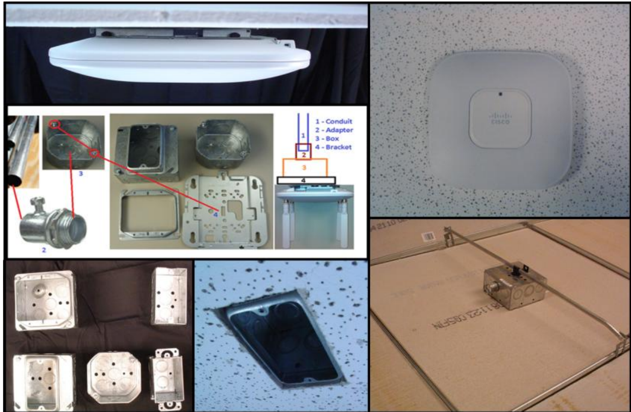
Figure 30: Installation of an AP onto an Electrical Conduit Box
